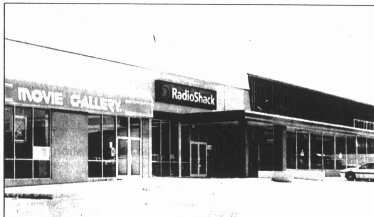
Radio Shack, a mainstay in Big Spring Mall for about 15 years, has relocated to the old Winn Dixie building just west of the V'al-Mart Supercenter. Radio Shack joins Movie Gallery and Dollar General, leaving just one space open at what was once Winn Dixie. Radio Shack Manager Bill Conner said the store is a little bigger at 2,500 square feet and has been remodeled. The store moved on July 6 and reopened at its new location on July 7 and is having several in-store specials this weekend as part of its move.
