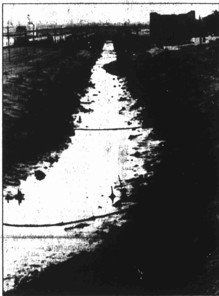
The newly expanded channel on Beals Creek is shown in this photo shot looking west from the Benton Street Bridge.
