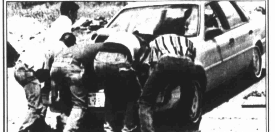
M & M Ditching employees help a motorist get her car out of a ditch they had dug across Wasson Drive. She crossed through the cone barrier and drove into the ditch thinking she could get across.
