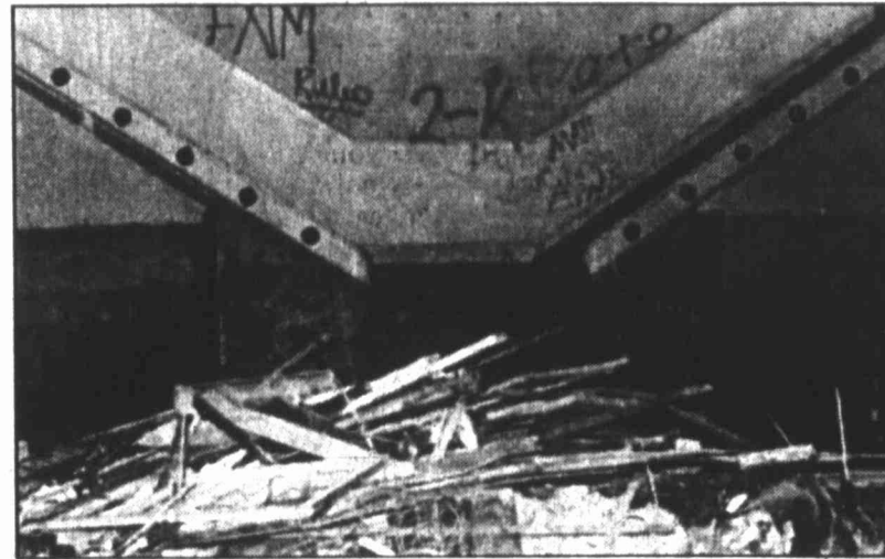
The same view of the staircases to the Settles Hotel ballrooms taken 69 years apart. All that remains of the split staircase is a metal frame while the lobby floor is piled with rubble.
