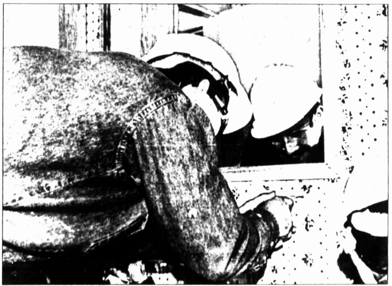
Paul Endtricht puts one of the finishing touches of the first home to come out of the Signal Homes plant in Big Spring.
