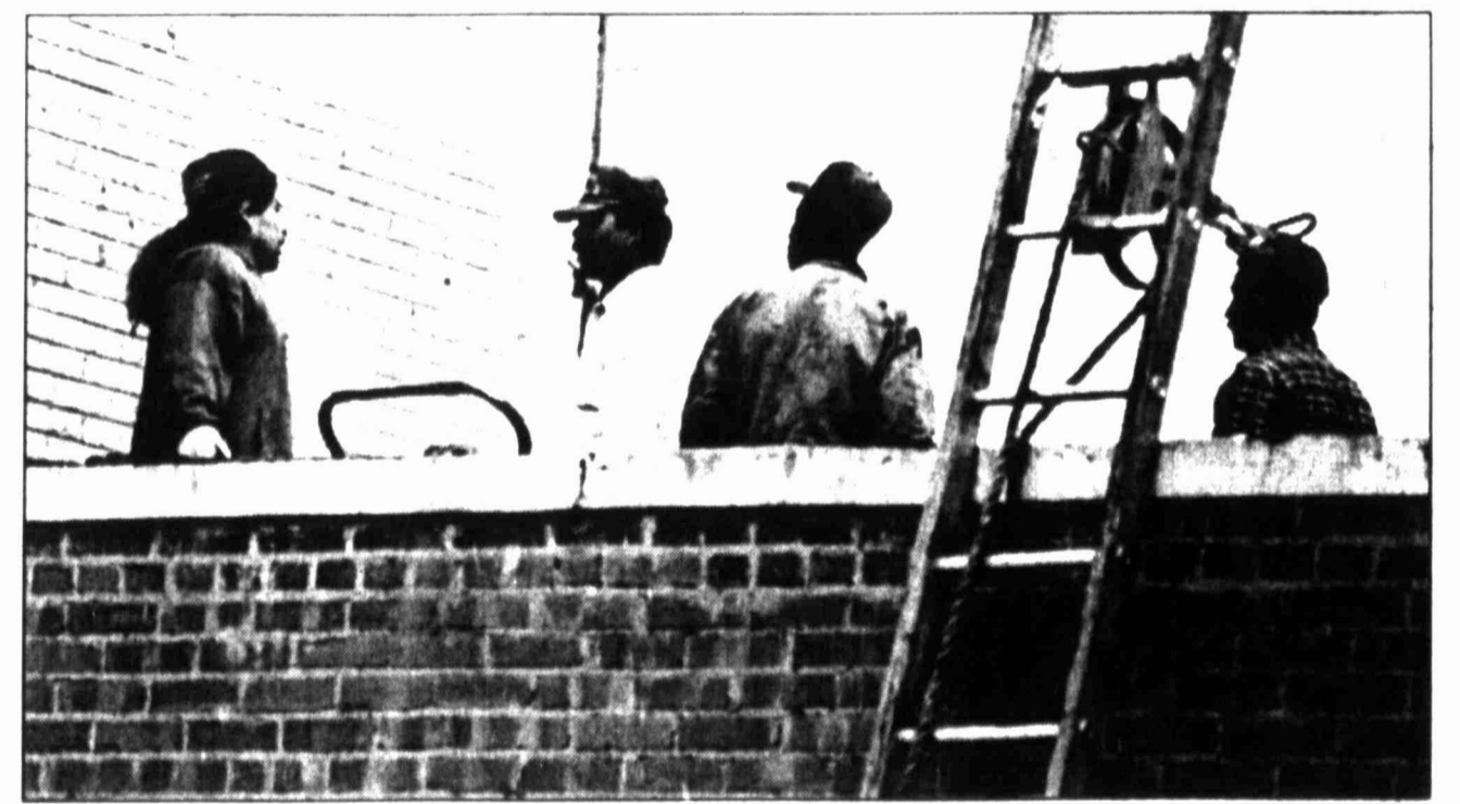
The Boy Scout Center remodeling effort is nearing an end. Wednesday afternoon, this group of workmen put finishing touches on the roof.
