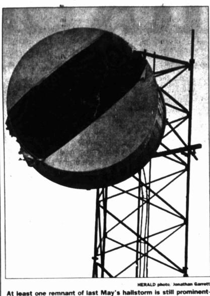
ly displayed over the downtown area. The cloth cover over this transmission tower, located due south of the Southwestern Bell building on Runnels, was ripped during the May 10 storm and still hangs in shreds.
