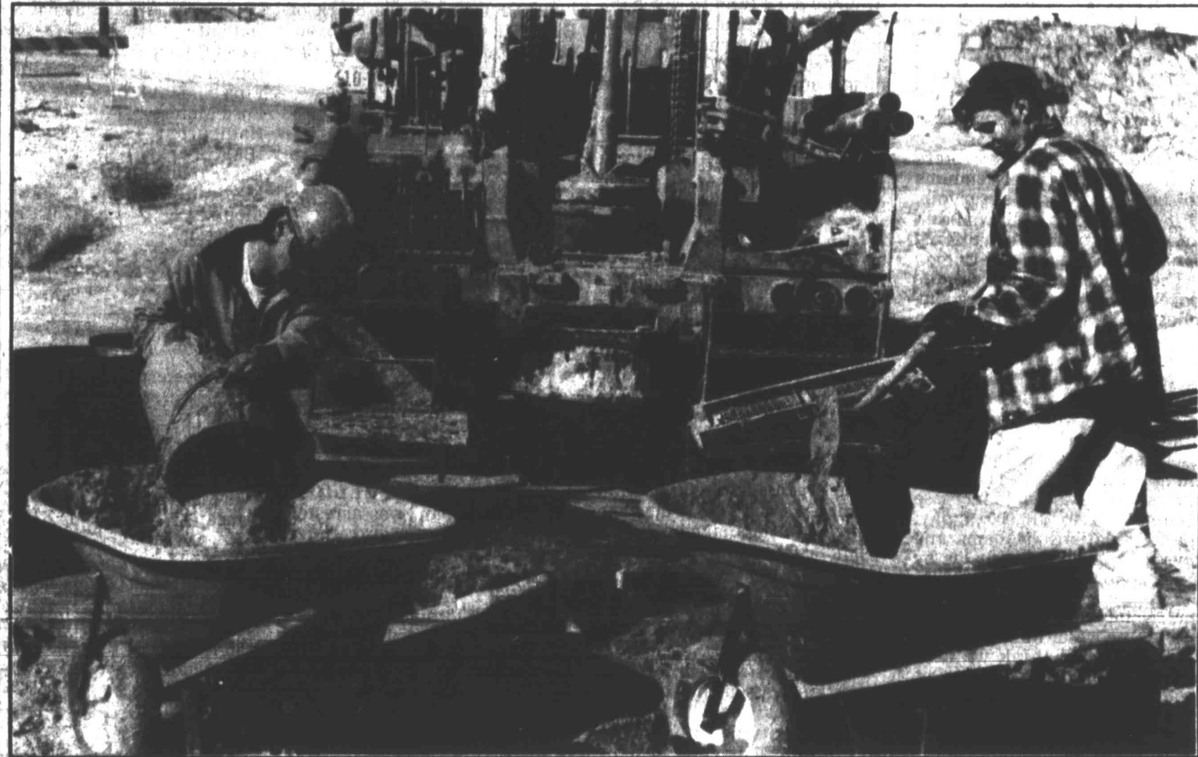
John Lynch (left) and Scott Williams begin an environmental sight assessment at Eighth and Gregg Streets. They will be drilling four wells until they hit ground water which, according to Williams, should be about 55 feet down. They will then return in a few days to take samples.
