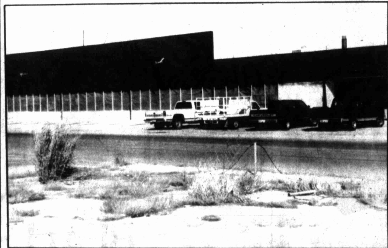
Remodeling and construction continues on the old Gibson's and The Box building at 2309 Scurry. The giant refurbished building will become the new home of Elrod Furniture in early 1997.
