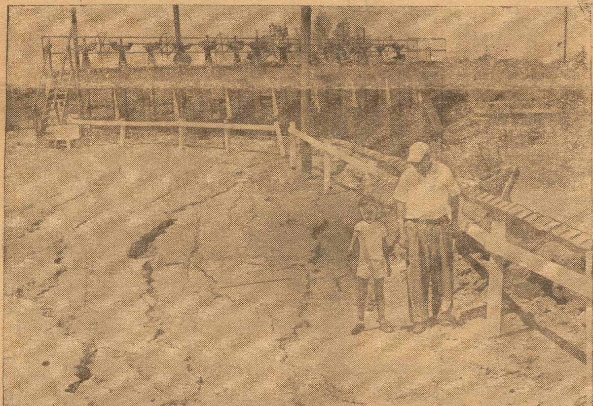
EARTHQUAKE CRACKS EARTH NEAR CANALS . . . A man and boy inspect the cracks in the earth near an irrigation canal near Calipatria, Calif. One day recently two severe earthquake shocks were felt by residents in the town. As a result of the shocks, buildings were damaged, windows shattered and bridges were knocked askew. The quakes caused the cracks in the canal. The man and boy are J. Bianco, Calipatria bank manager, and Mike Maracinni, 6. As a result of the quakes and in fear of new quakes, most all of the business establishments in the town were closed and practically all of the residents of the town have moved away temporarily.
