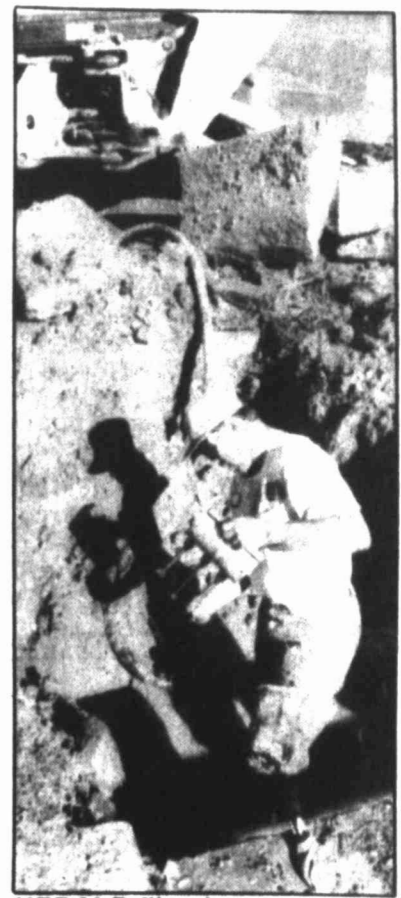
HERALD file photo A city worker repairs a water main break in this file photo. Workers will be busy this week replacing a 20-inch valve on a major transmission water main.
