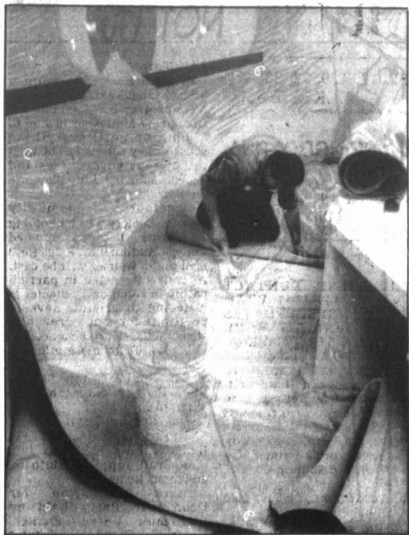
Miguel Rodriguez applies carpet adhesive to the floor of the new Big Spring City Council chambers Wednesday before setting the carpet into place. Along with the carpet, other interior work currently being done to the old downtown fire station includes testing of the sound system.
