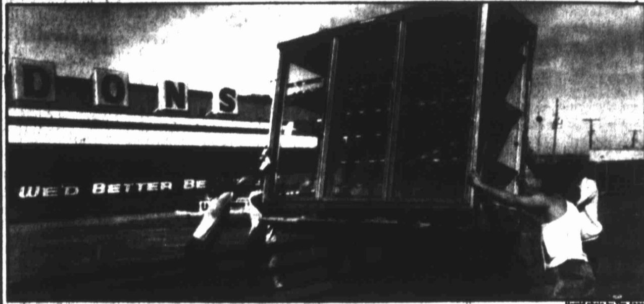
IGA workers guide a large freezer unit from the former Don's IGA Grocery onto a trailer Wednesday. Among the rumors circulating around town is one that the building will be remodeled into a medical facility.
