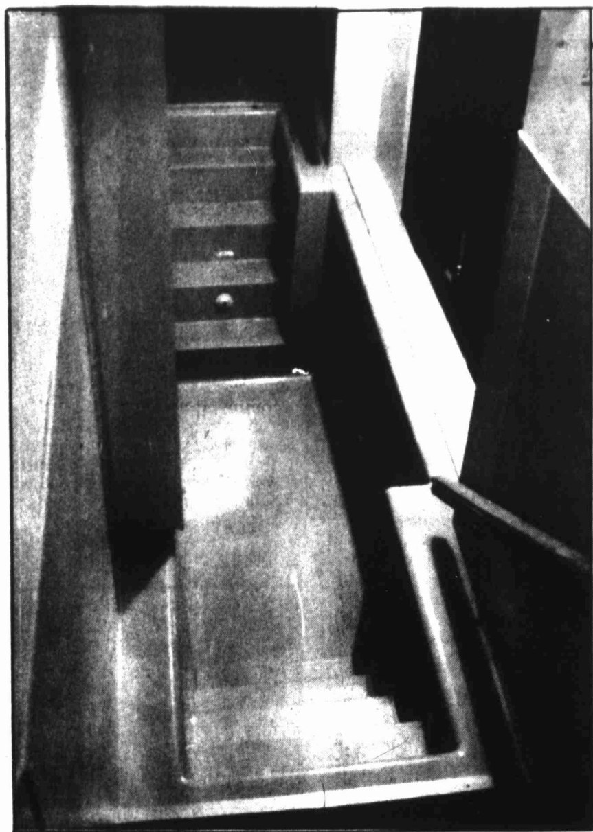
This $4,500 baptistry, installed in September, replaced the old copper tub in First Christian Church. Church secretary Christine Brockman said the old tub leaked so badly, those walking in and out of the tub could feel and hear the floor squishing.
