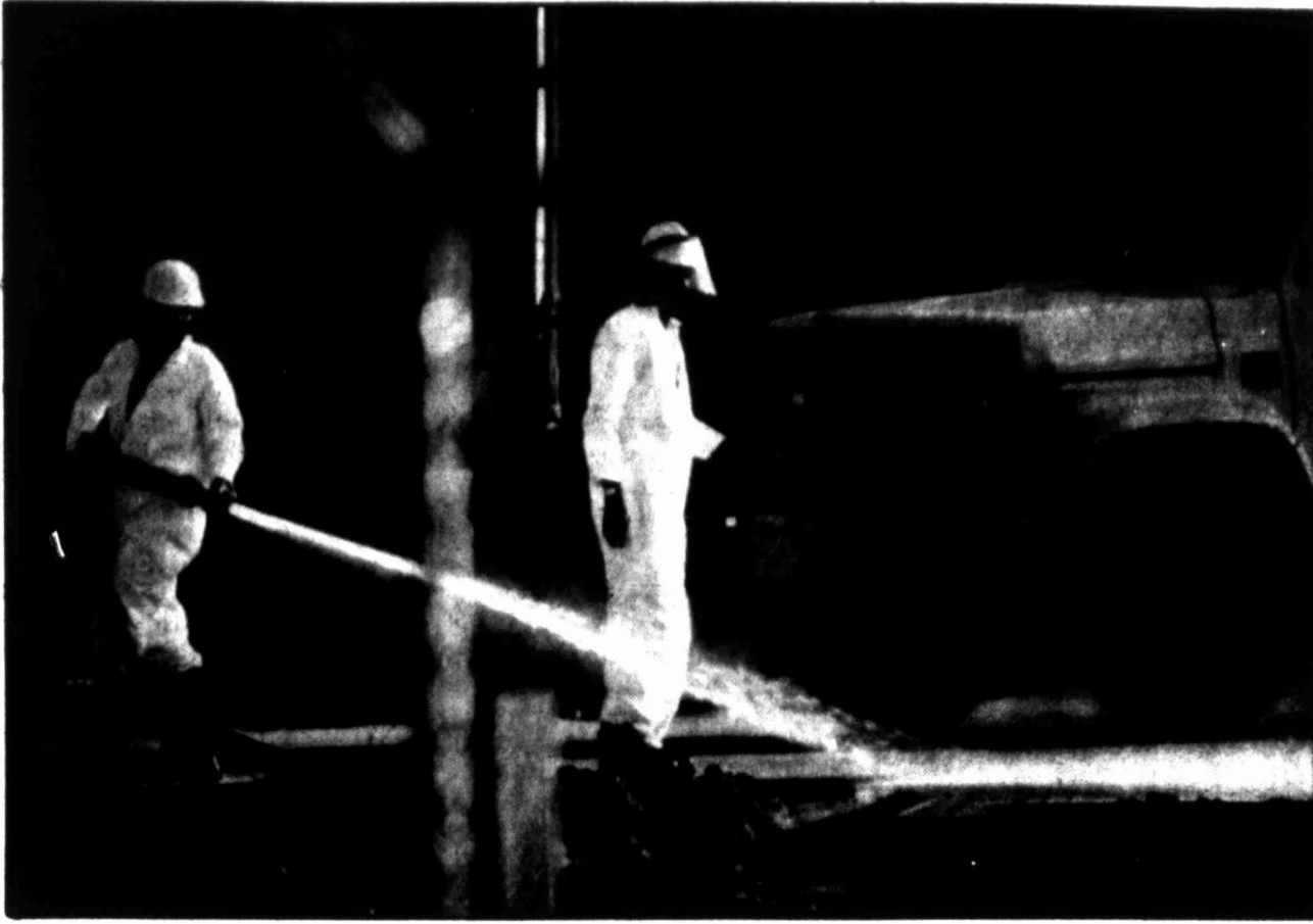
Cleanup crews wash arsenic-tainted soil from their equipment after a day of removing contaminated dirt from Commerce properties in this file photo.
