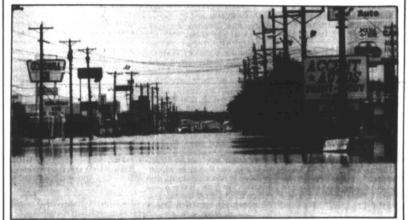
Flood waters from Elm Creek spread over much of the west side of Abilene on Saturday, including this portion of north First Street and Leggett Drive. The flooding is the result of heavy rains from the remnants of Tropical Storm Dean.
