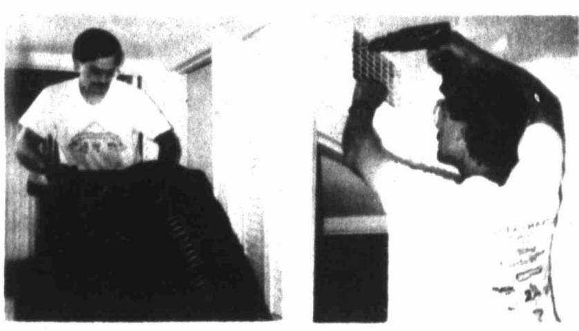
Mark Heinis prepares to clean, sanitize and seal a local air duct system.
