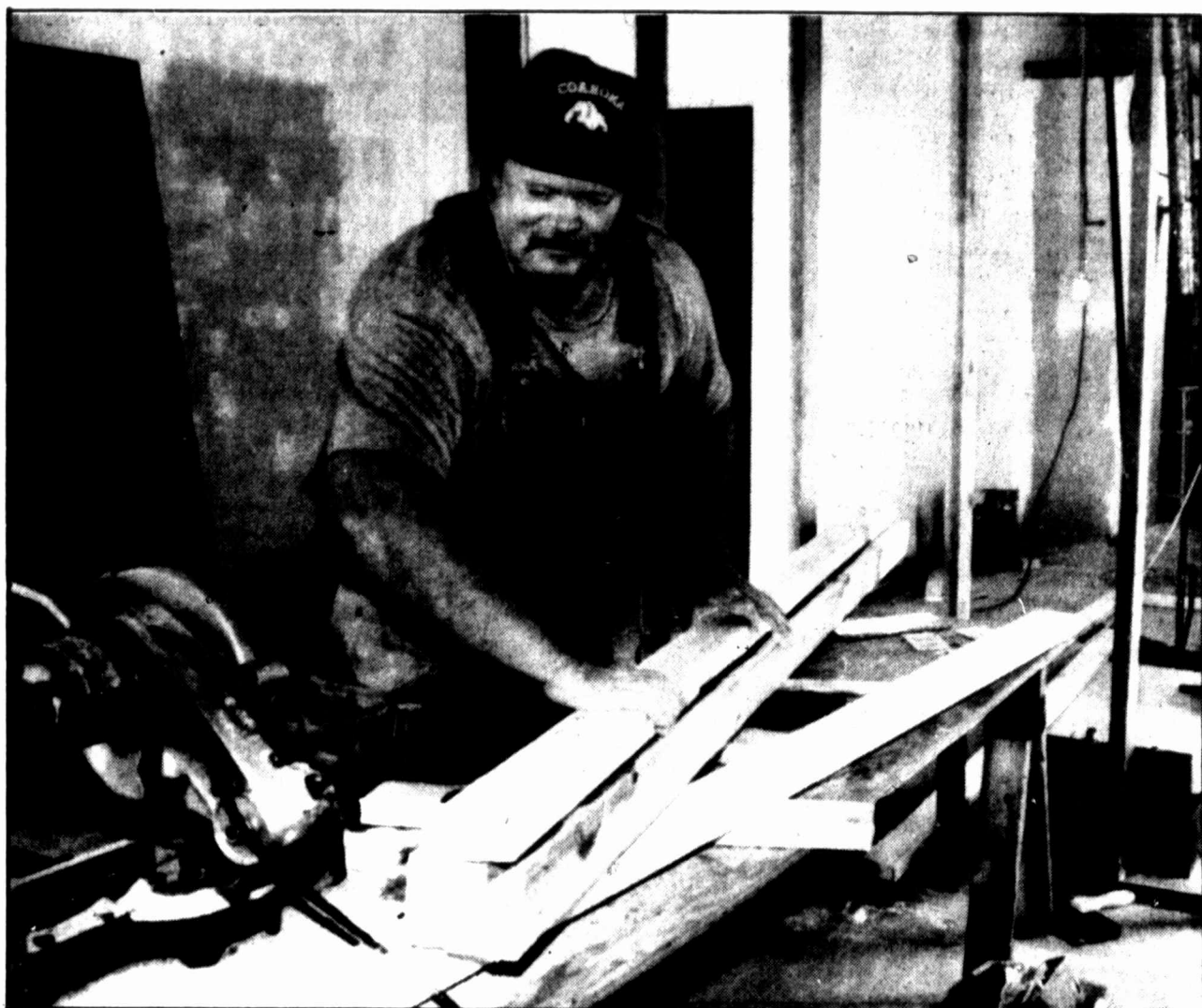
Hank Williamson prepares to work on wooden planks being used in the remodeling of a building at 1202 W. Fourth St. The building, scheduled to open May 1, will house nine families free of charge for a weekend when they come to visit relatives in the city or federal prisons.
