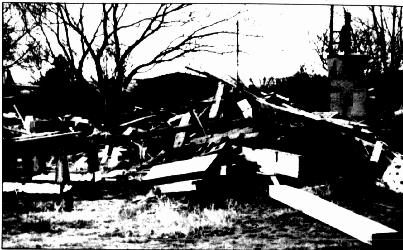
This lot next to Big Spring resident Glenda Low has her and several neighbors worried about the fire hazard and possible health hazards it poses. Low filed an official complaint with the Texas Natural Resources Conservation Commission in Odessa Monday that the lot has become an illegal dump site.
