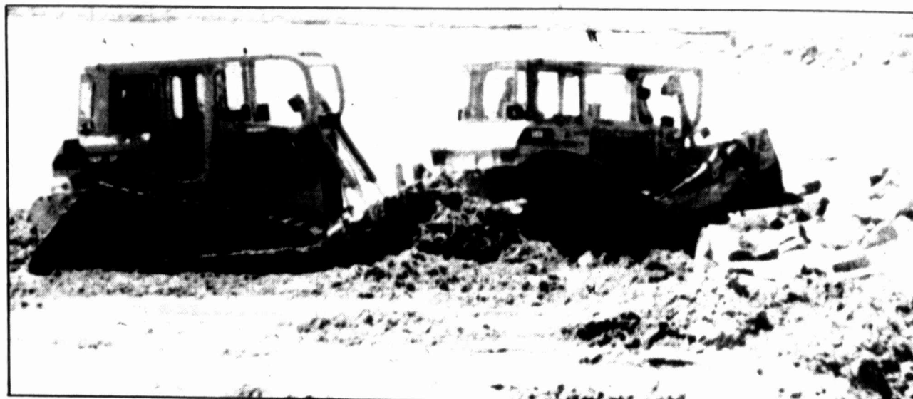
Bulldozers refurbish an eroded beach in Galveston. Work on the $5.9 million Beach Nourishment Project began two months ago, a year after residents voted to raise the sales tax to fund it.
