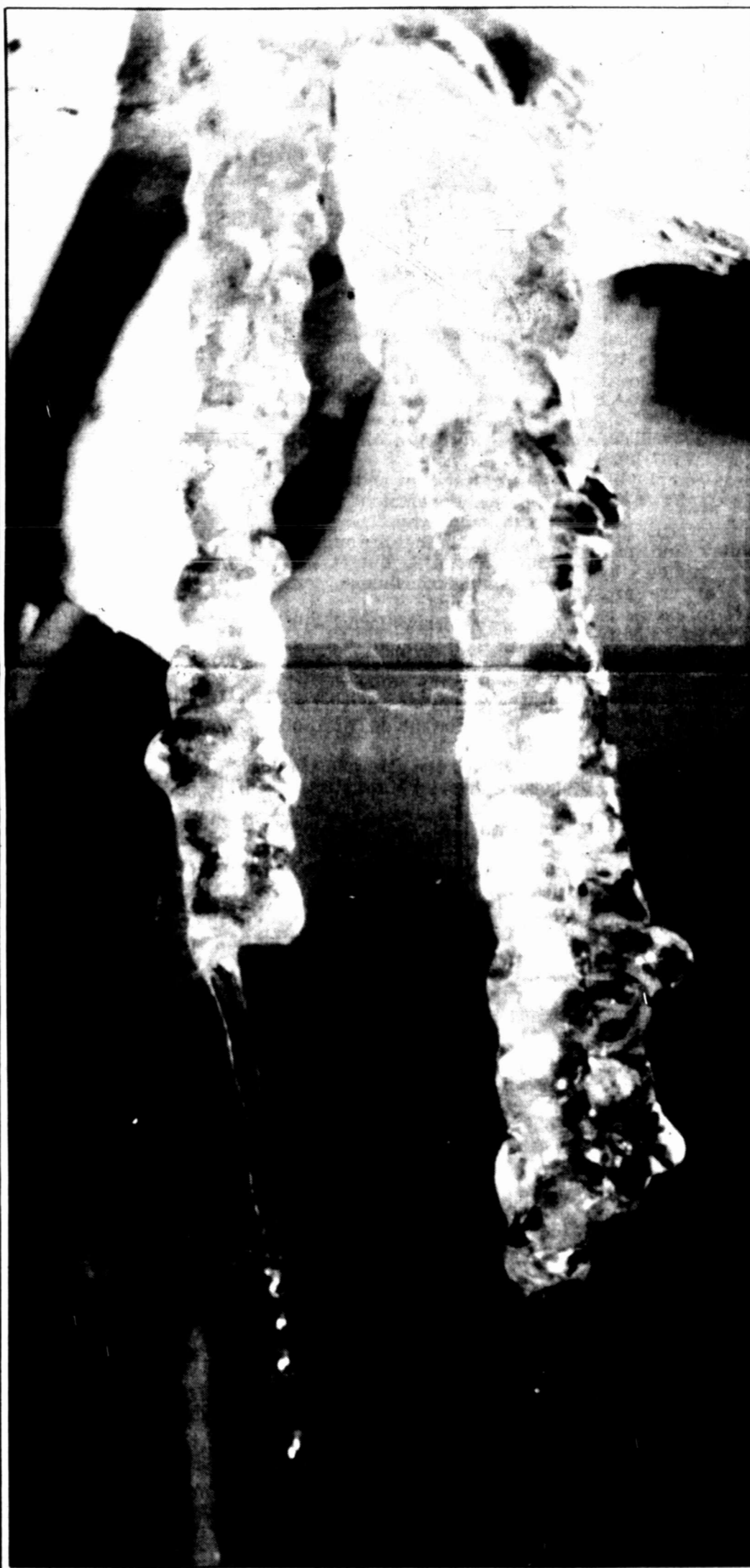
Water drips from icicles that hang from the roof of a home Friday as warmer weather settled back in the Big Spring area for the weekend. By Saturday, all traces of the week's cold weather had vanished. However, cold weather has returned but not as viciously. Low tonight expected to be in the lower 20s.
