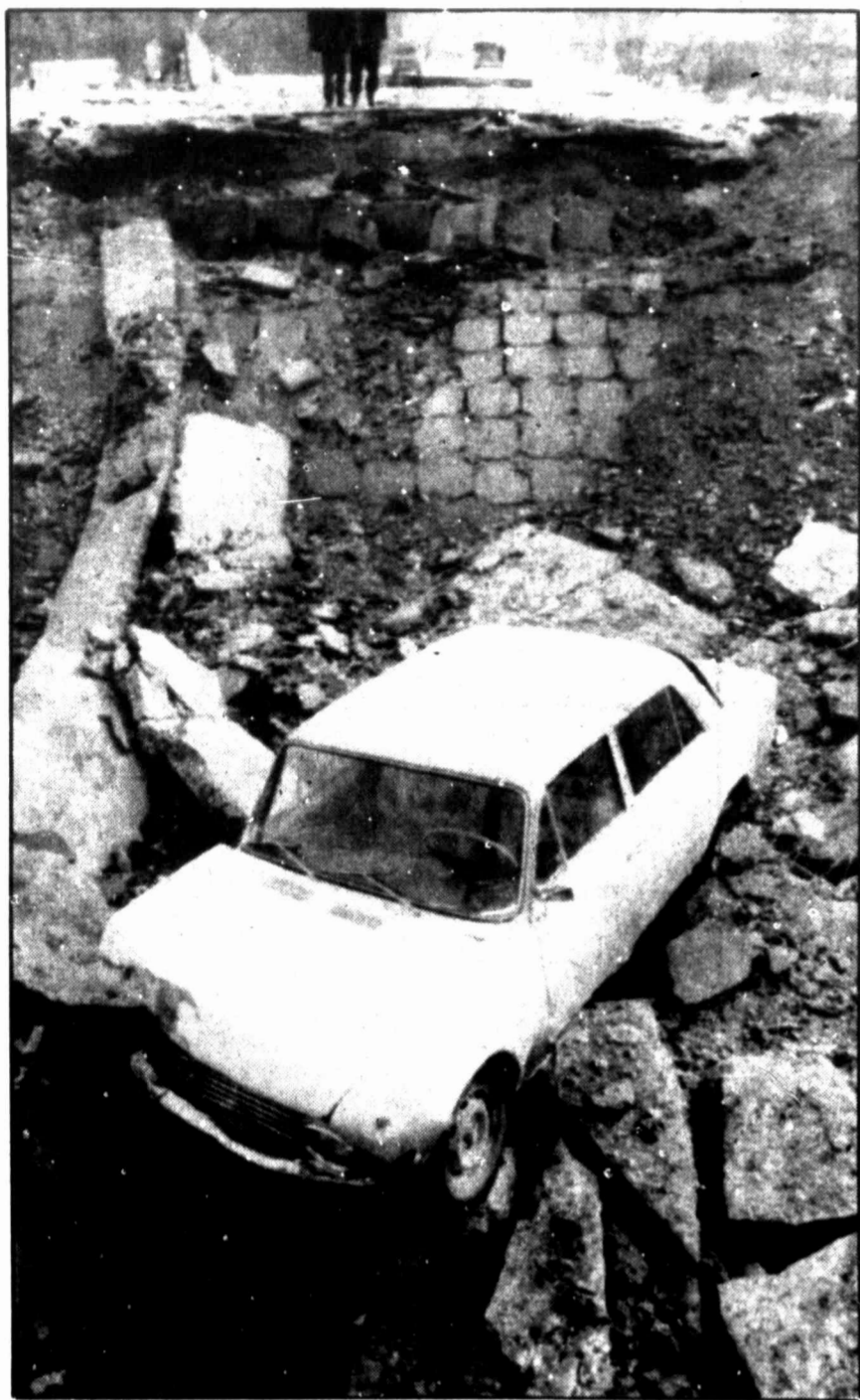
The wreckage of a car lies among the debris of a bridge, blown up overnight some 12 miles west of Grozny Saturday. The damage forced refugees to pass through a stronghold of Chechen forces opposed to rebel leader Dzhokhar.
