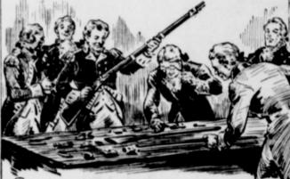
IN THIS FACTORY MASS PRODUCTION -INTERCHANGEABLE PARTS - FOUNDATION STONES OF MODERN INDUSTRY AND TODAY'S NATIONAL DEFENSE WERE BOTH DEVELOPED BY ELI WHITNEY .- BY 1806 HE PRODUCED 10,000 MUSKETS WITH EACH LOCK. STOCK AND BARREL INTERCHANGEABLE.
