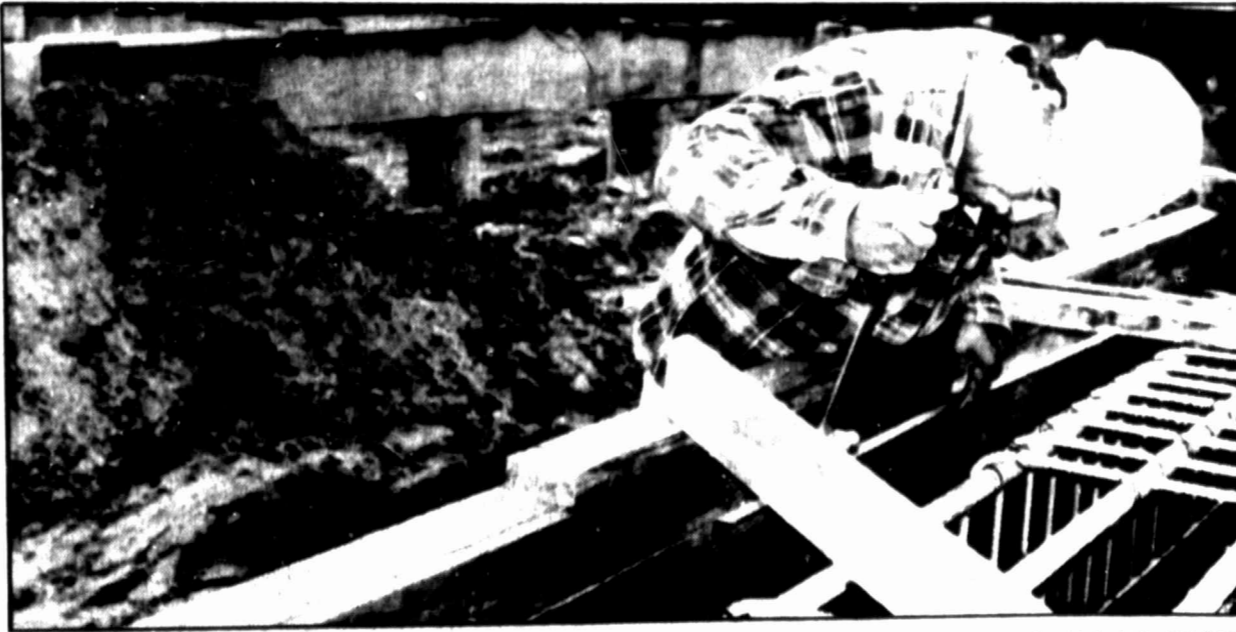
Jesse Franco nails a small guide board into place as he was constructing a form for the concrete that will be a new support on the I-20 bridge widening project recently.
