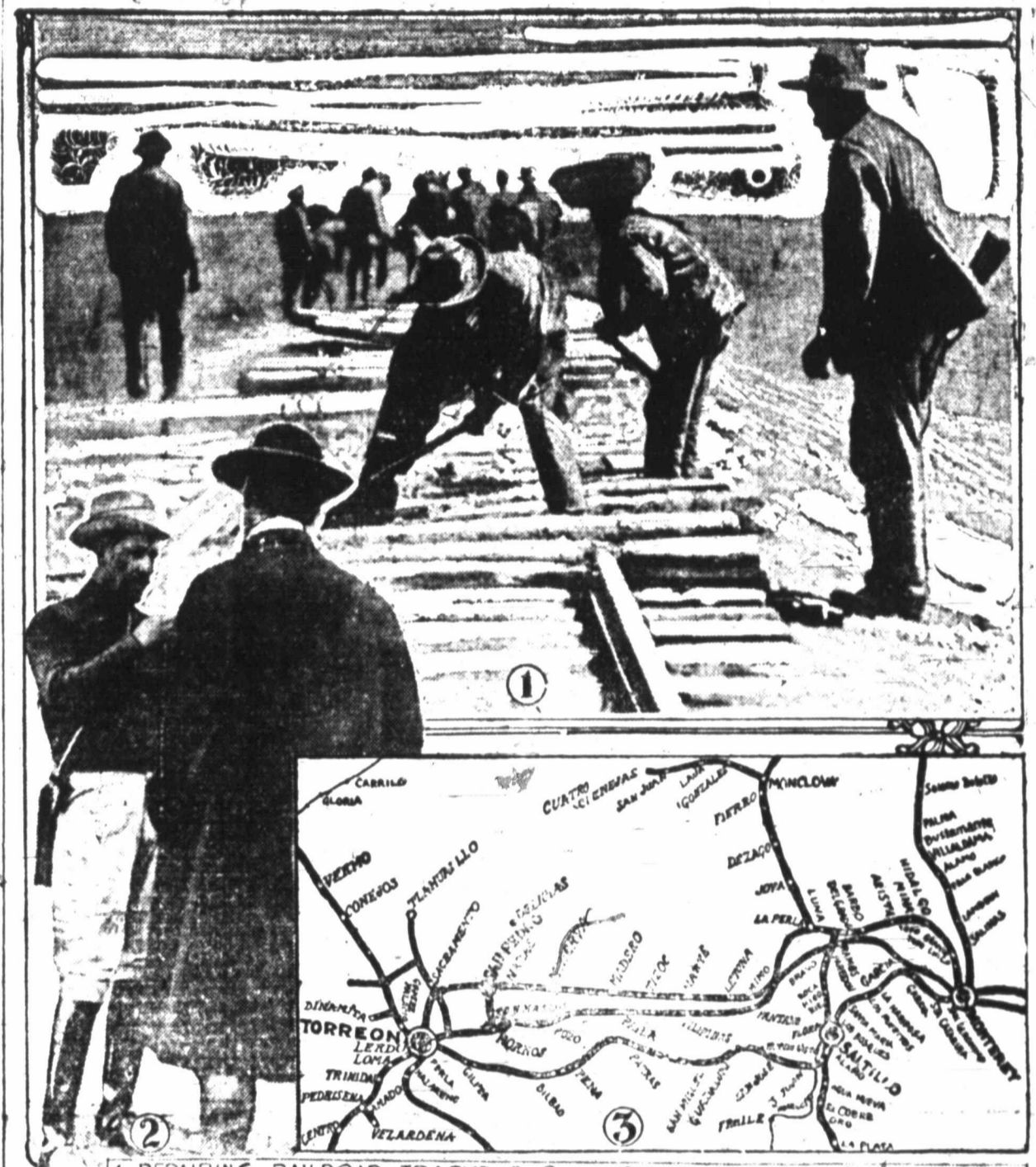
1-REPAIRING RAILROAD TRACKS, 2-Gen. ANGELES, 3-CENTRAL FIGHTING ZONE
