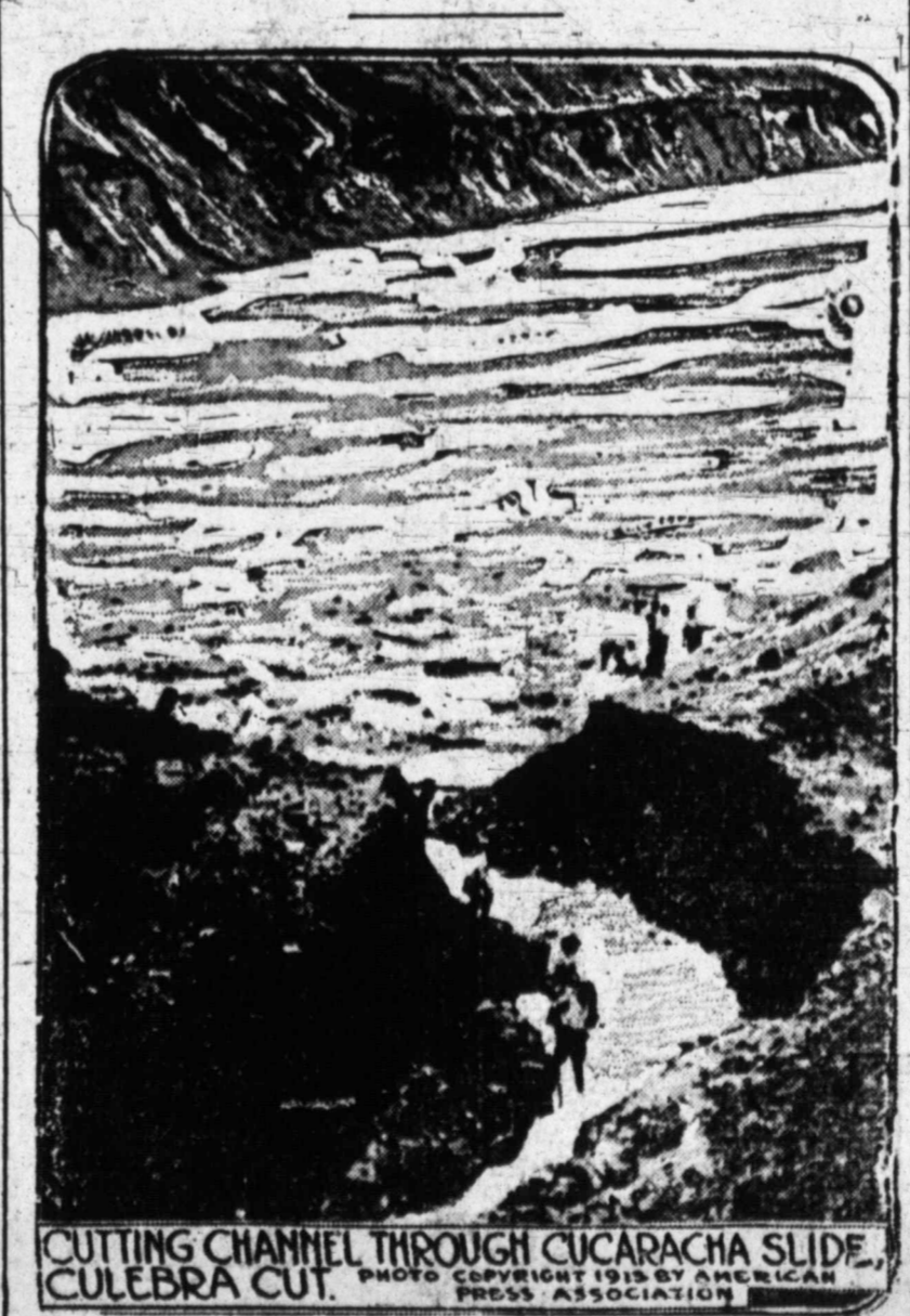
CUTTING CHANNEL THROUGH CUCARACHA SLIDE, CULEBRA CUT. PHOTO COPYRIGHT 1913 BY AMERICAN PRESS ASSOCIATION
