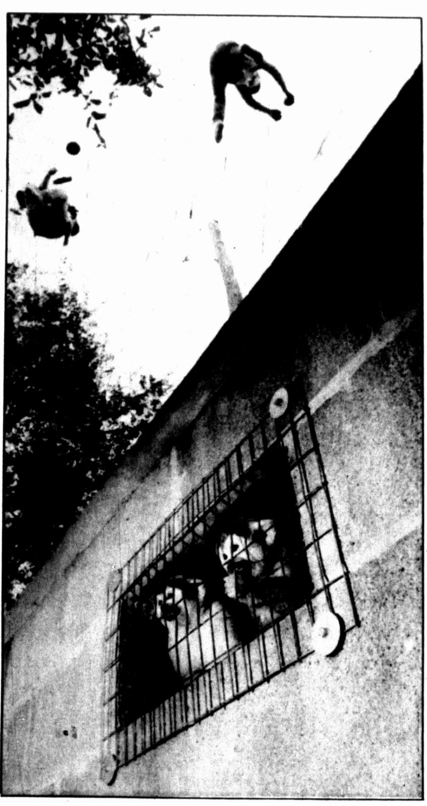
Carolyn Tatulinski, left, and Wayne Rider work above as spider monkeys look out a small opening in their cinderblock habitat at Primarily Primates, a wildlife refuge near San Antonio. The Southwestern Bell telephone employees were stringing cable and wire to build a bigger, more natural living area for the monkeys.
