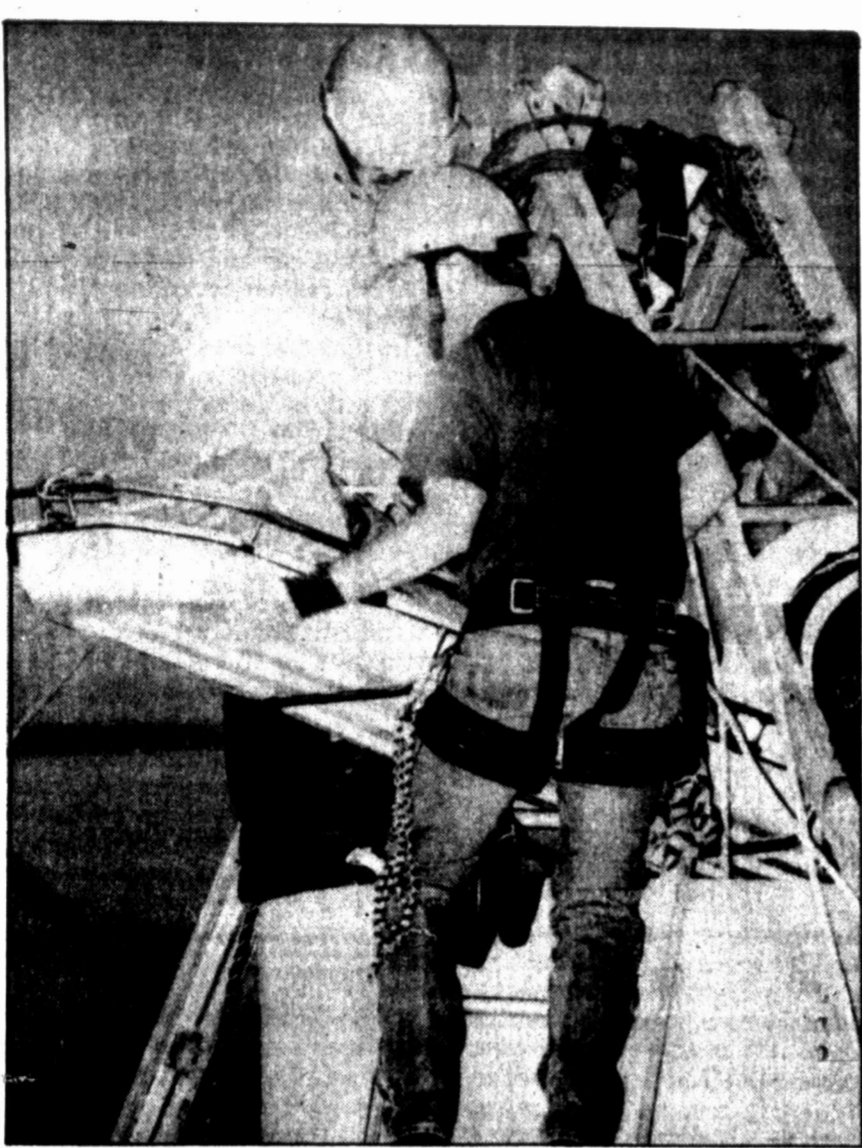
Rescue personnel lift the body of Carroll Gene Davis of Fritch from a water valve at the Amarillo Regulating Reservoir Thursday. Davis' body was retrieved about 200 feet from the channel's reservoir entrance where he was clearing debris from the intake structure.
