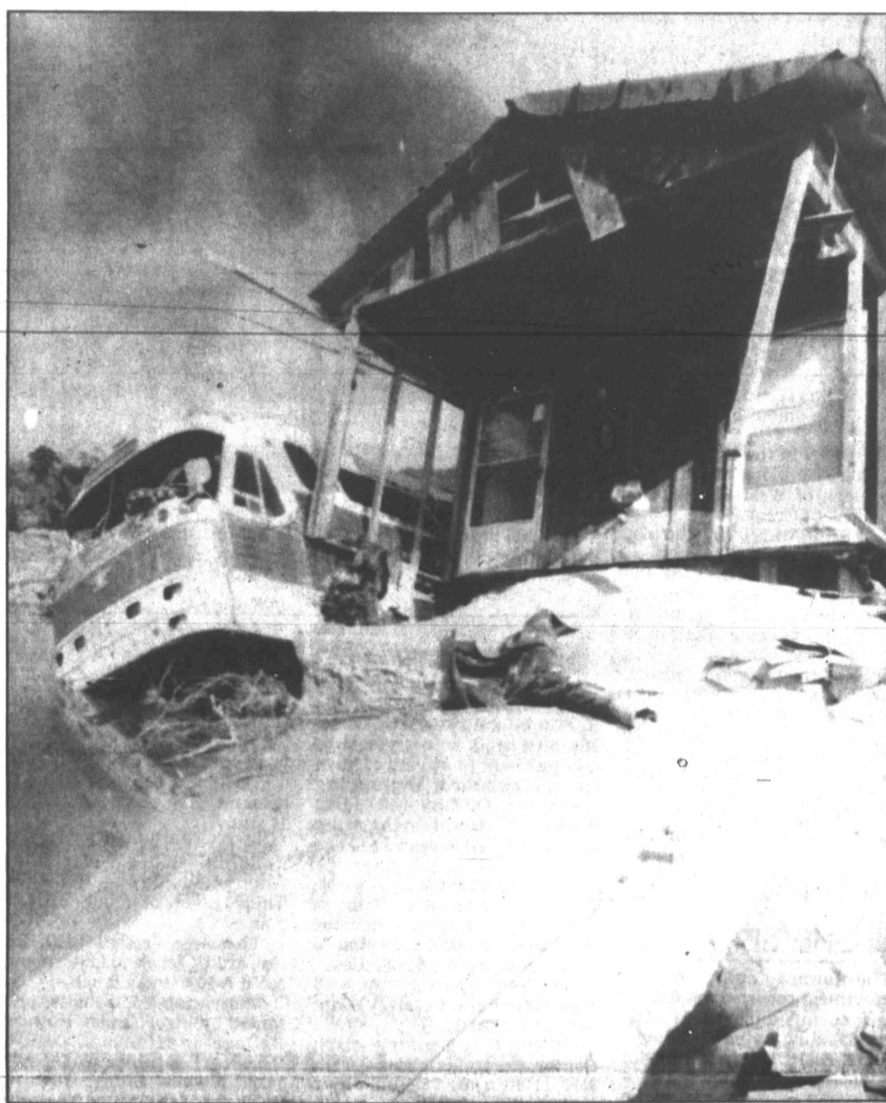
A bus that was crushed by a collapsing boat house along the San Jacinto River in Harris County was found Monday. The house fell due to the floods that poured through Southeast Texas, killing 19 people. See related story page 3.
