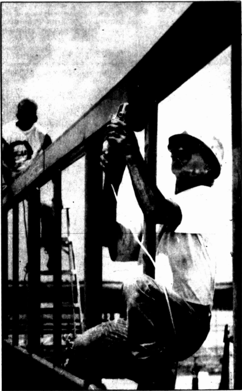
Tom Ragsdale stands on the handrail to grind weld joints smooth as construction work continues on the new Mid-Tex Detention Center at the Big Spring Airpark Wednesday afternoon.
