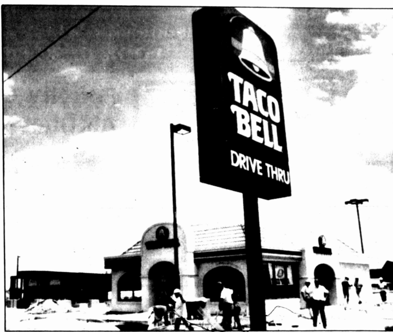
Workers continue construction on the Taco Bell restaurant location. Taco Bell, specializing in Mexican food, plans to open the facility soon.
