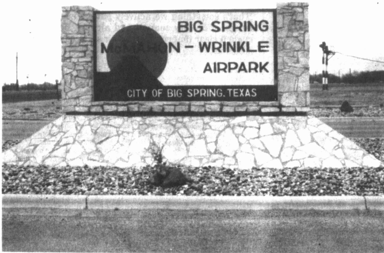
The Big Spring McMahon-Wrinkle Airpark is a drawing card in the city of Big Spring's efforts to bring industry to this area. The airpark is home to many different and varied industries who have taken up residence in the old Webb Airforce Base buildings.
