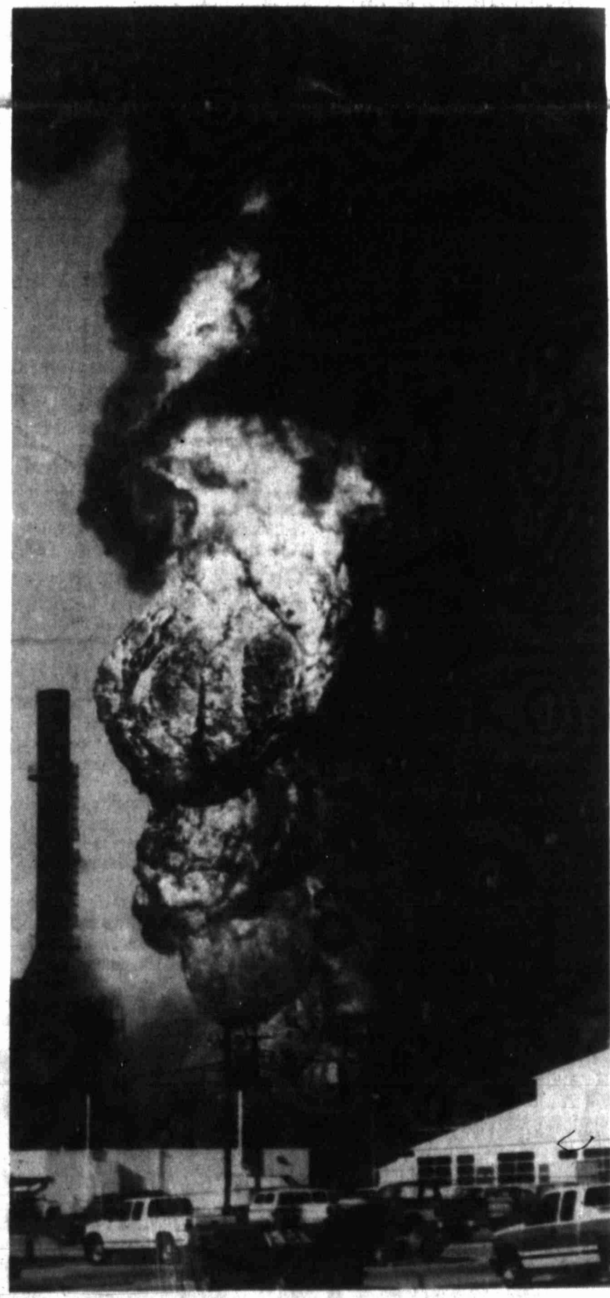
The March 3, 1993, fire which caused millions of dollars of damage to a Fina Refinery reformer unit. It took only six weeks for repairs to be completed and to get Fina back up and running at full capacity.
