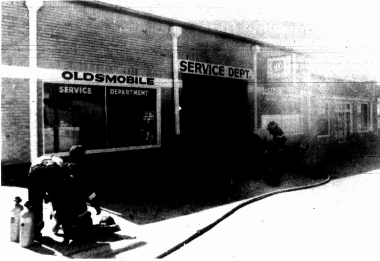
A fire at Shroyer Motor Company service department Thursday resulted in $25,000 in smoke damage and no injuries. It was caused by a vehicle gasoline tank ignited by a broken bulb.
