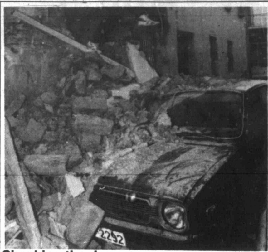
Checking the damage
