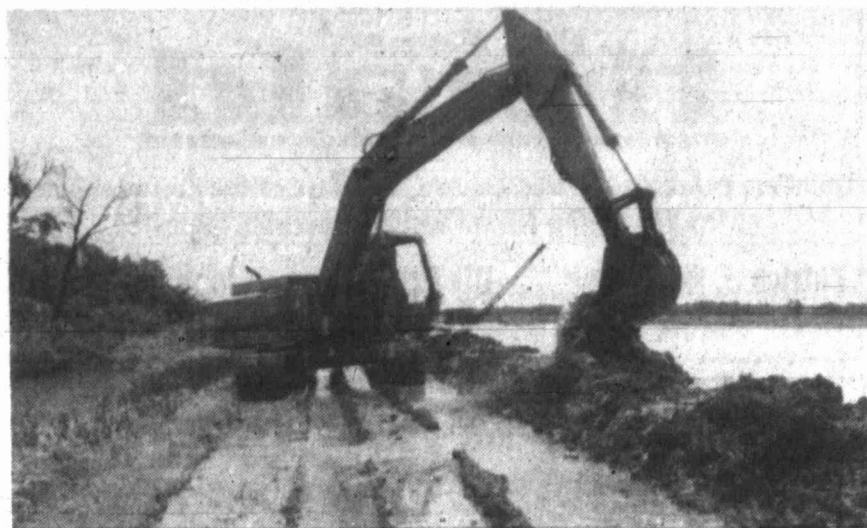
Dennis Showalter makes a desperate effort to shore up a levee with an excavator along the Tarkio River near Craig, Mo. Tuesday in a bid to save a nearby family farm. The swollen river began breaching and topping local levees in northwest Missouri Tuesday and is expected to flood thousands of acres Wednesday. Showalter's attempt proved to be in vain.
