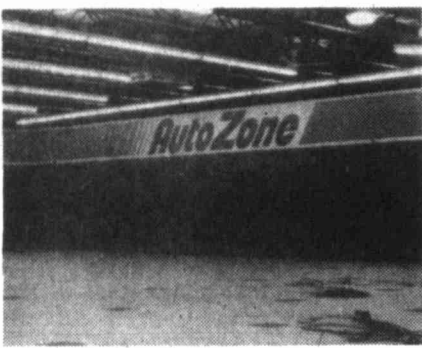
Construction on the AutoZone store at Second and Gregg is nearing completion. The auto-parts store is expected to open in three weeks, a construction foreman said.
