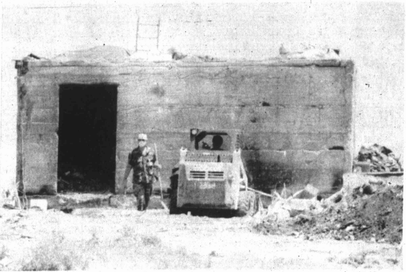
Investigators clear debris from the area in front of the concrete blockhouse at the destroyed Branch Davidian compound near Waco Monday. Independent arson investigators supported FBI claims that members of the cult started a fire that consumed their compound.
