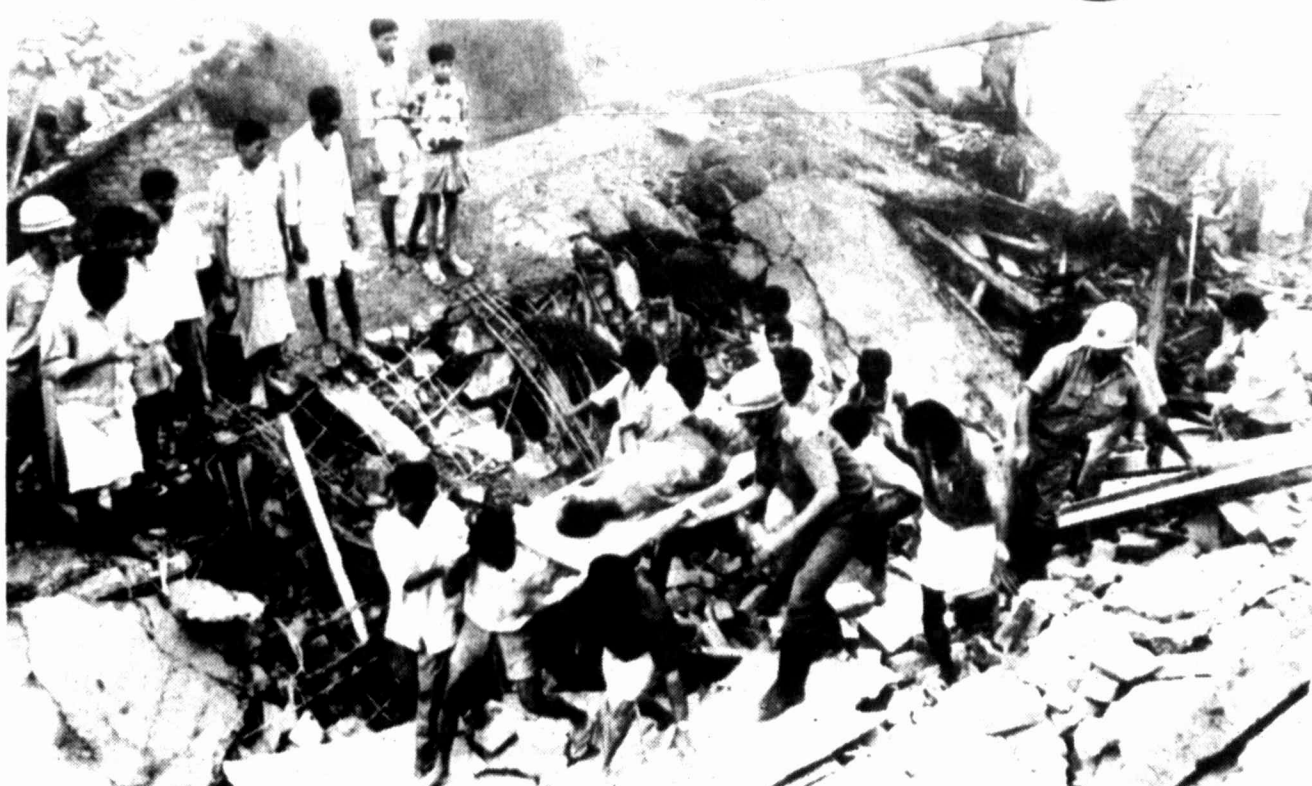
Firefighters and local residents aid in the recovery of bodies from the collapsed buildings in central Calcutta Wednesday. A huge bomb blast rocked the congested area earlier in the day, killing 50 people and injuring about 100 others.
