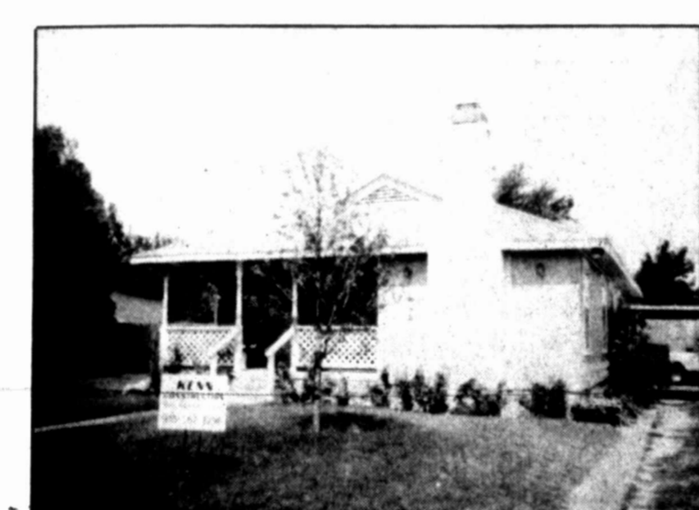
Roofing, painting & remodeling are all part of Kenn Construction's forte. They offer complete remodeling services and free estimates.
