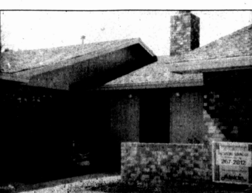
Pictured above is another fine American home by Big Spring Siding Company. Spring is just around the corner, so now is a good time to take a good hard look at your home exterior or overhang.
