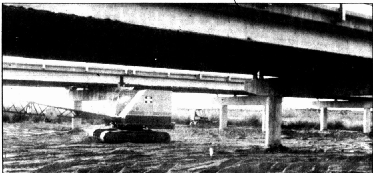
Construction has begun on two bridges northwest of Big Spring. The bridges comprise Interstate 20 as it crosses the Sulphur Draw area. Rebuilding the bridges, replacing deck plates and adding safety shoulders, should take about a year.
