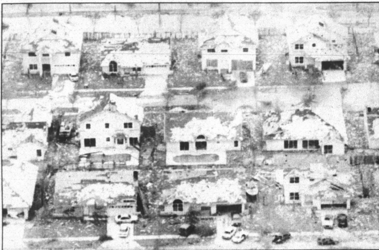
Rows of damage houses between Homestead and Florida City sit in the aftermath of the worst hurricane to hit the south Florida area in 60 years.
