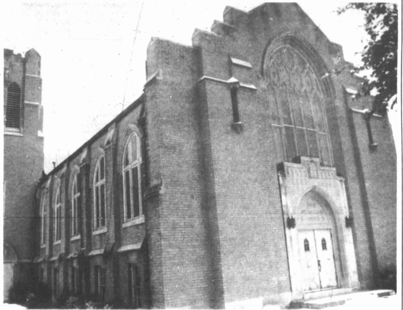
First Presbyterian Church is beginning a major renovation later this month. As part of the plan, this entrance on Seventh Street will be renovated to be more accessible to people with disabilities.
