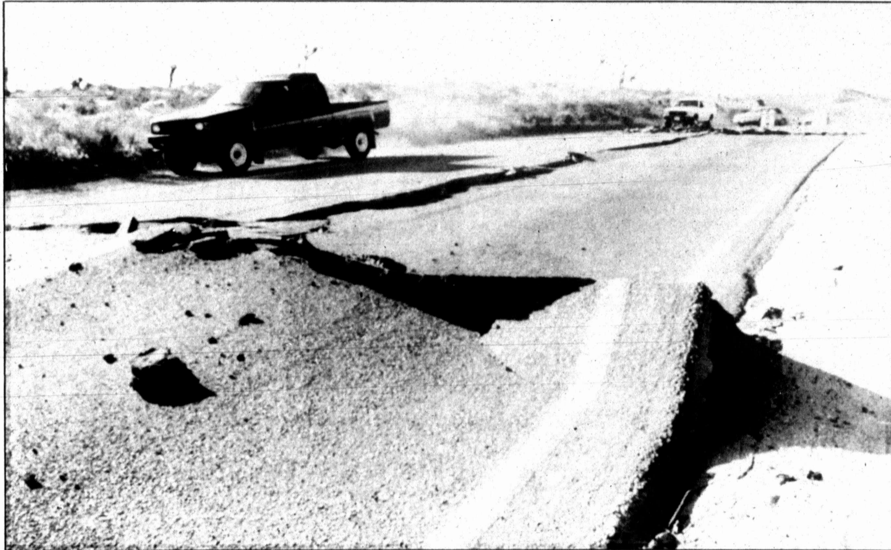
Vehicles are forced to drive on the dirt shoulder of California Highway 247, also known as Old Woman Road, in Yucca Valley, Calif., after an earthquake registering 7.4 on the Richter Scale buckled the roadway Sunday. More earthquakes hit the western United States early today.
