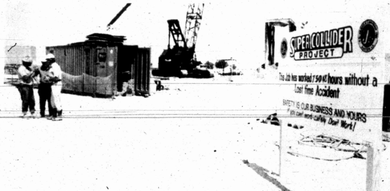
Construction workers stand at the site of the first shaft for the underground superconducting super-collider near Maypearl Thursday morning. The
