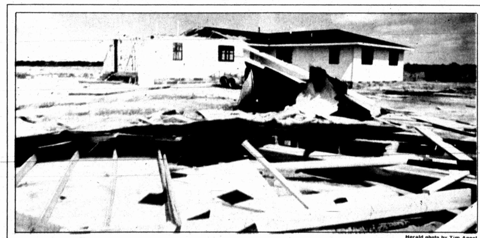
Storm damage An unoccupied, newly-built home on Jill Road, southwest of Coahoma, sits surrounded by debris after a suspected tornado struck the building Thursday evening, destroying the garage and part of the roof. A mobile home located on the same road also was demolished in the storm. For additional photos, see Page 5A.
