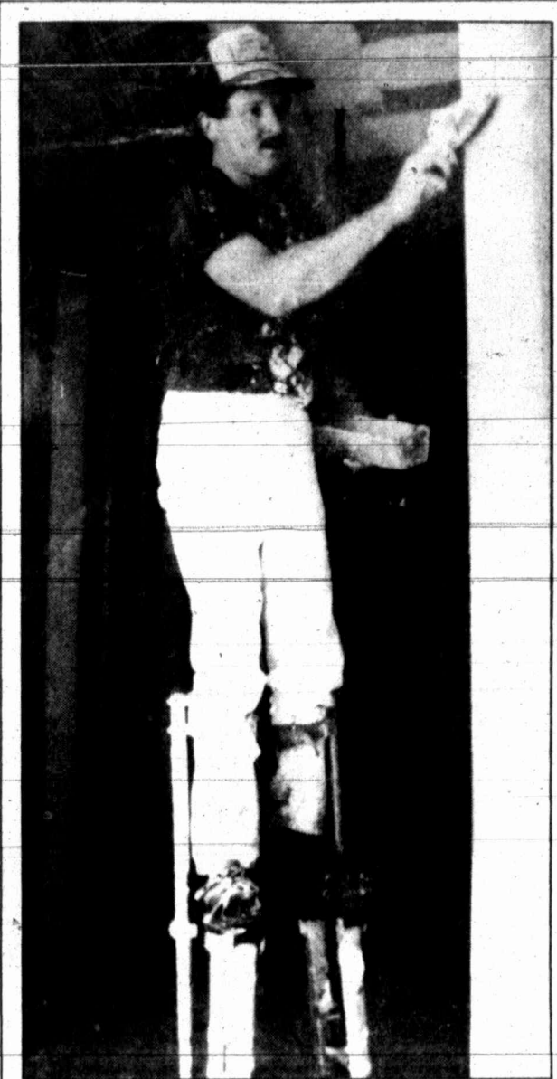
The long of it Standing atop stilts, Donald VanStory applies plaster to one of the walls in the new Activities Building at the Big Spring State Hospital Wednesday afternoon. The building is scheduled for completion at the end of August. Herald photo by Tim Appel
