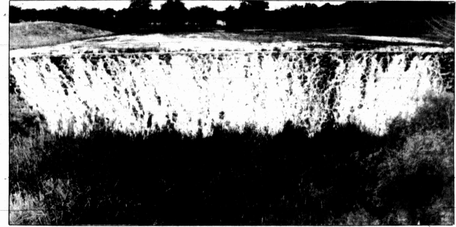
Water spills over the top of a dam at Comance Trail Lake this morning. More than one inch of rain fell on Big Spring late Monday, causing flooding on several Howard County roads.
