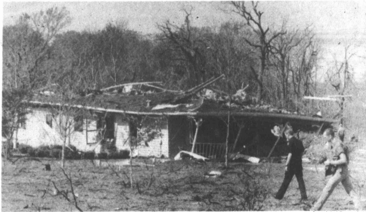
Department of Public Safety workers walk in front of a house that was rocked by a gas pipeline explosion Tuesday morning near Brenham. One person was confirmed dead and at least 18 were injured.
