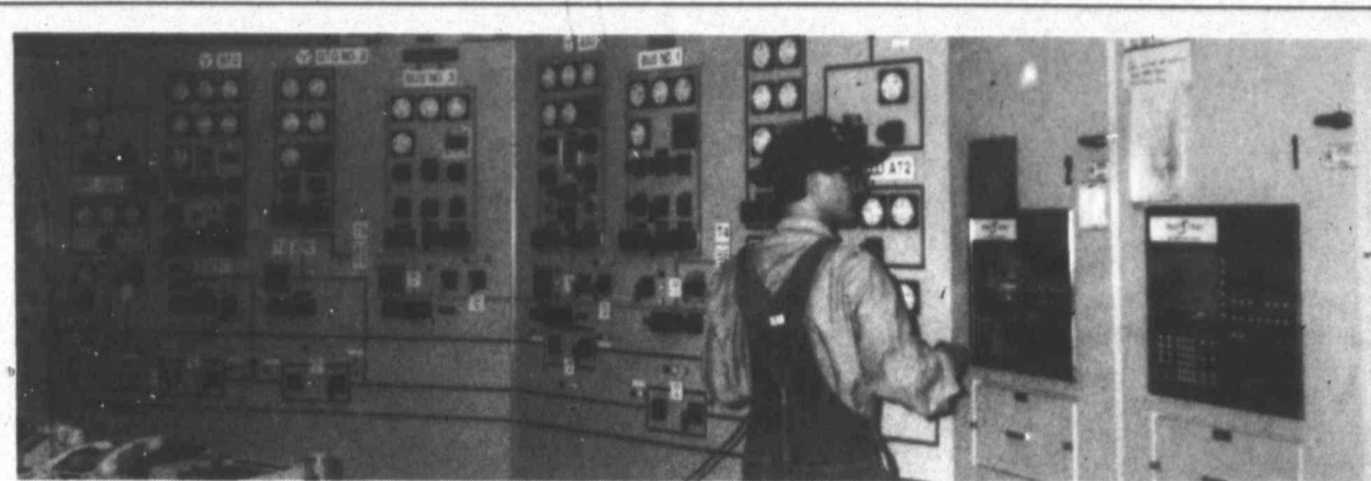
A control room operator monitors the daily operations in the Distributor Control System room at Power Resources Inc. located east of Big Spring, which last year received a tax abatement on more than $3 million in plant improvements. The plant produces electrical and thermal energy in the form of steam.
