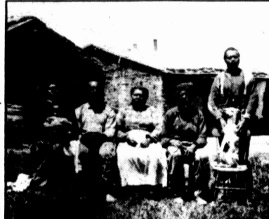
A family in front of their sod house in Nebraska in 1887. Since there were few trees on the plains, many people built their first homes of sod (a layer of soil, held together by roots.)
